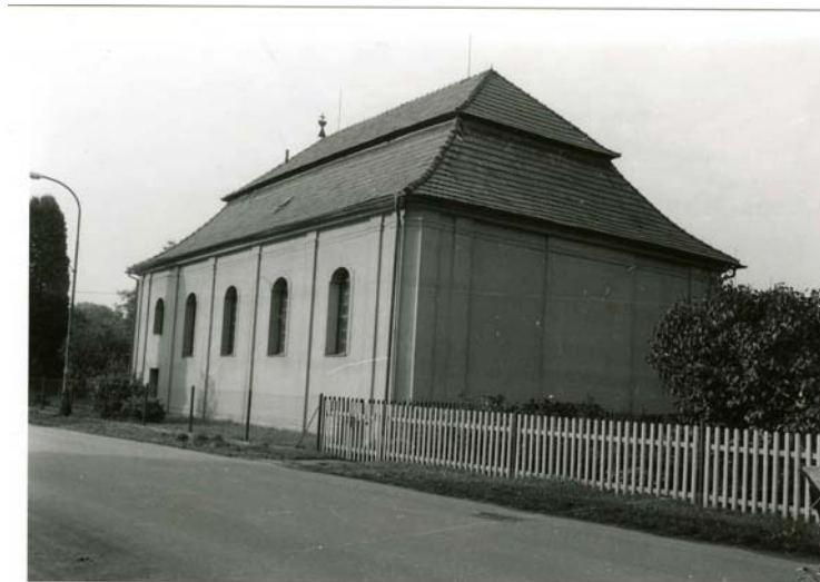
Synagogue after alterations for the Czechoslovak Hussite Church (view from south-east).
