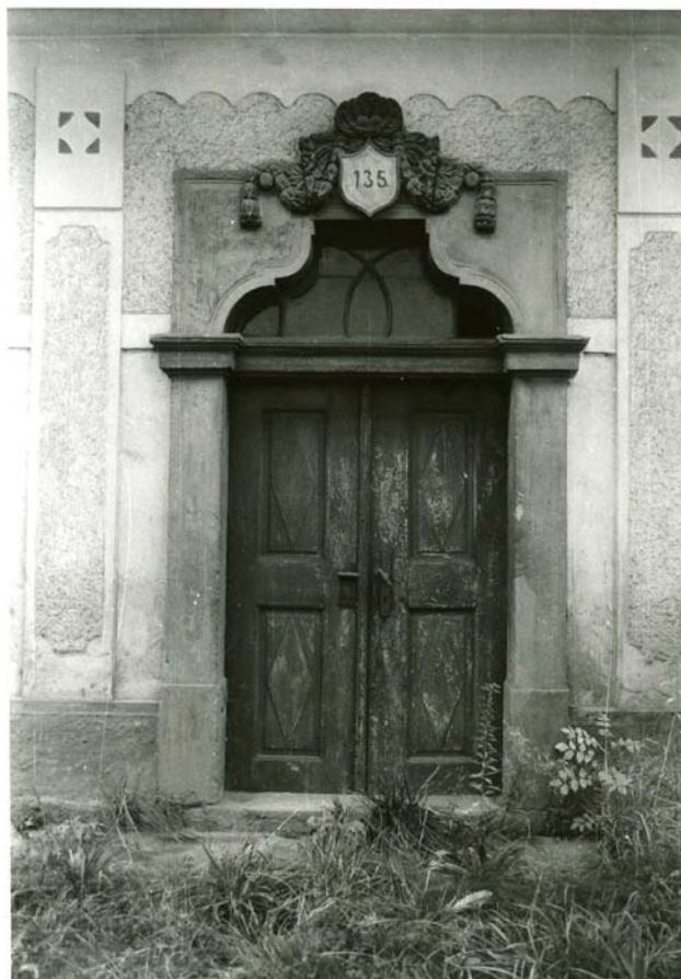
Portal of house no. 135 (originally no. XXIX, belonging to the Fanta and Agular families) in Švermova street.
